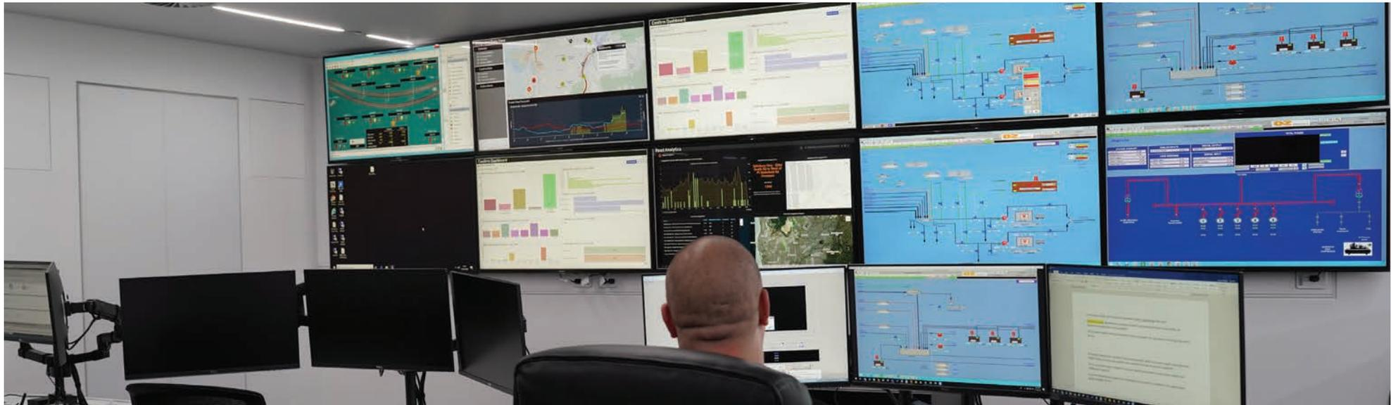
SAGE's National Operations Centre (NOC), based in Adelaide, supports clients to remotely resolve faults and improve their uptime. The RSM enables fast connection with the NOC in times of need.
